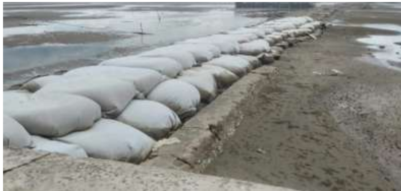
Figure 5. Erosion-Control Geobags from the PHKT CSR Program
