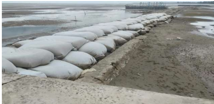
Figure 1.1 Geobags for Coastal Erosion Control
